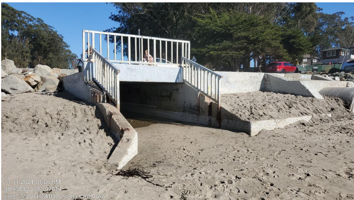
Photograph 10. View of Moran Lake Beach and the box culvert beneath East Cliff Drive, facing northeast. November 11, 2021.
